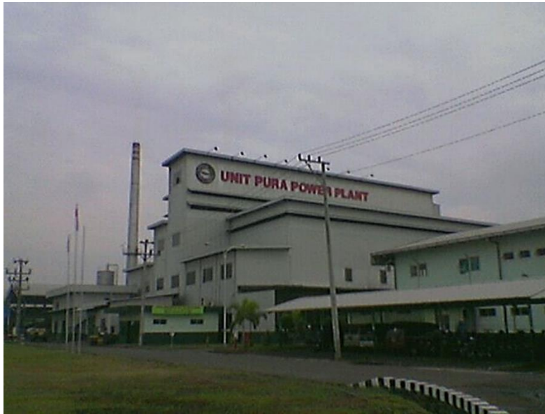
Foto 1. Unit Power Plant PT. Pura Barutama Kudus
