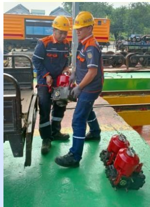
Gambar 1. 1 Pemindahan distributor valve manual
